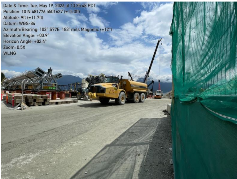
Photo 10. One of two water trucks observed actively operating.
