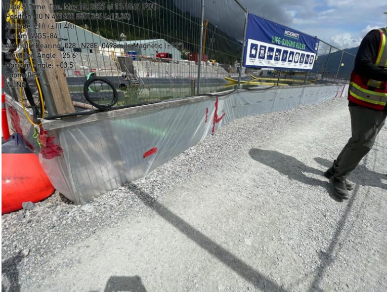
Photo 8. Poly exclusion fencing secured to metal fencing around perimeter of water treatment ponds.
