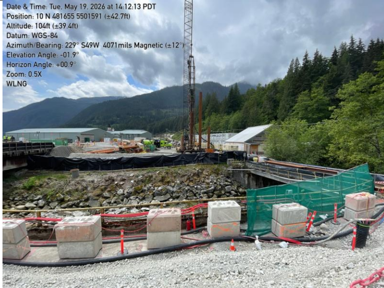
Photo 11. Erosion and sediment controls along side Mill creek pile driving activities.
