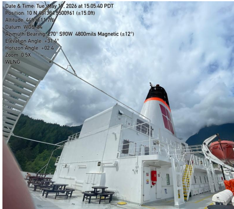
Photo 13. Exhaust stack from Floatel 2.
