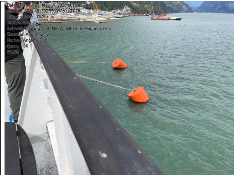
Photo 3. Two anchor points installed off stern of vessel.
