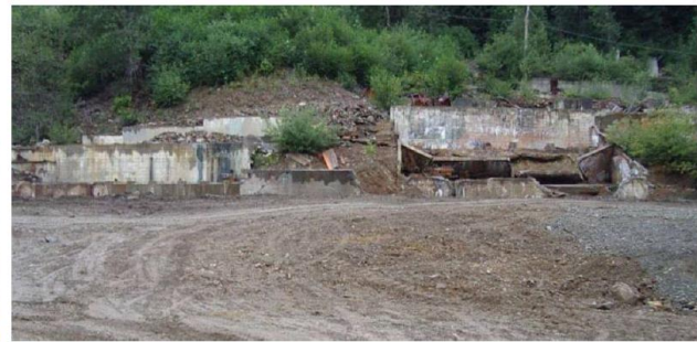
Mill Site After Clean-Up
