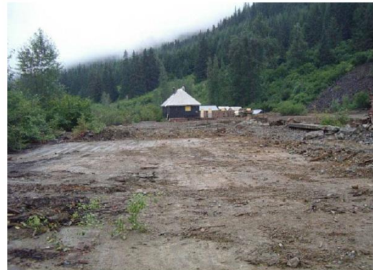
Mill Site After Clean-Up
