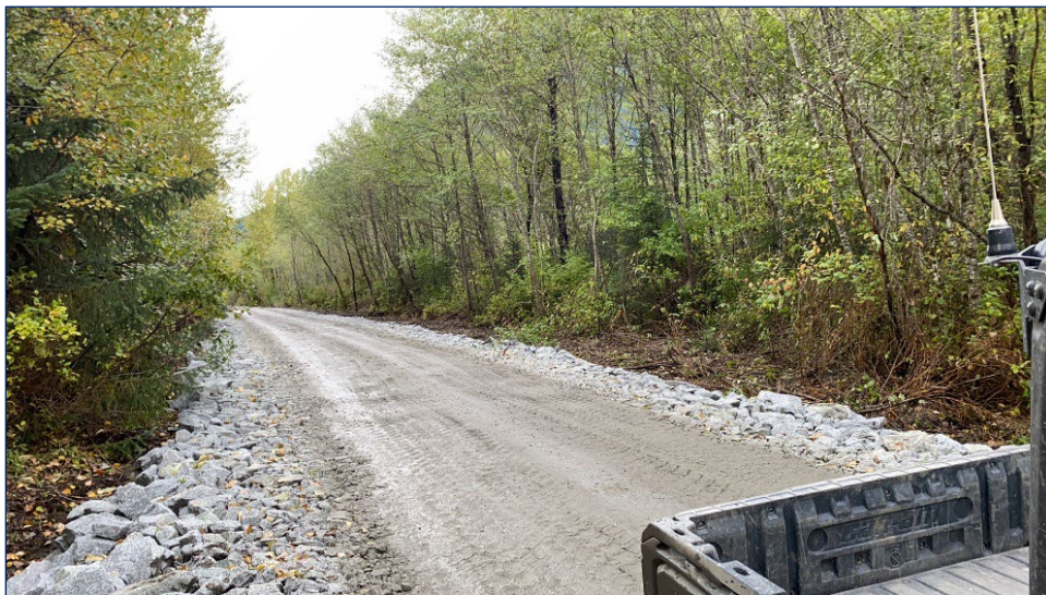
FIGURE 4-8: BALLASTING OF ACCESS ROAD, SEPTEMBER 2024
