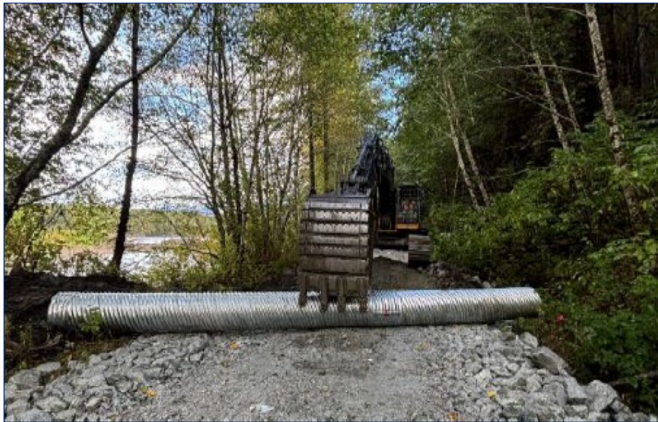
FIGURE 4-4: ACCESS ROAD CULVERT INSTALLATION, SEPTEMBER 2024
