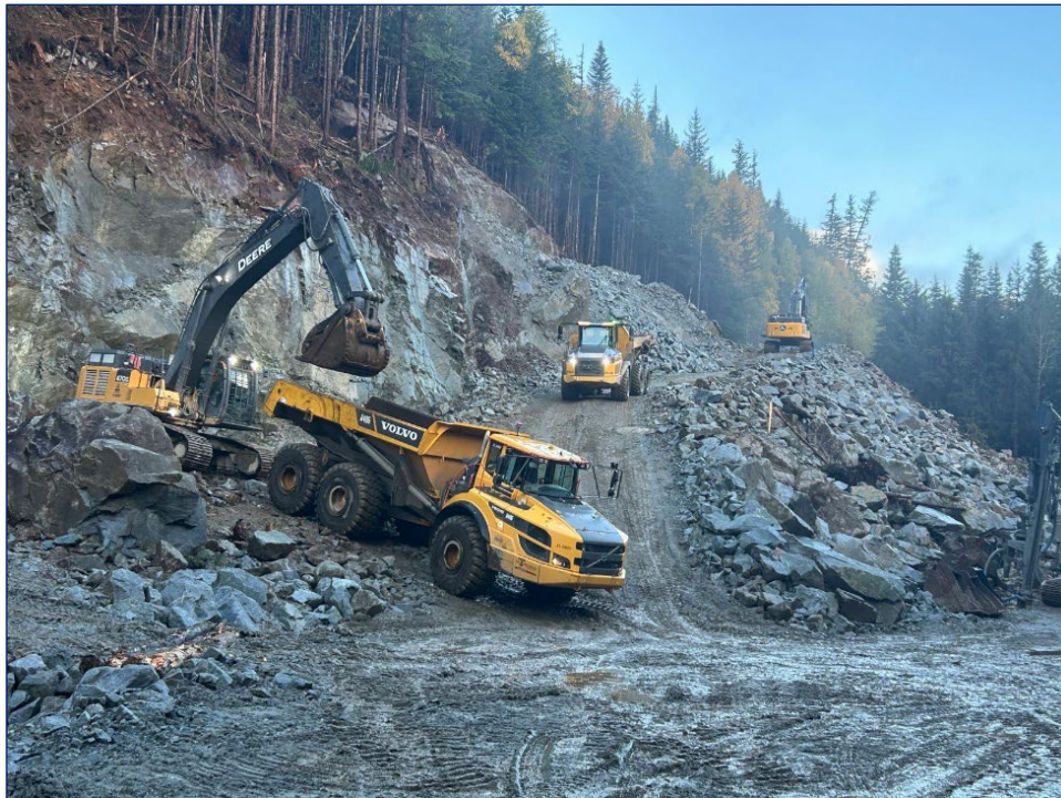
FIGURE 4-12: LOADING TRUCKS AT BORROW PIT (1 OF 4), SEPTEMBER 2024
