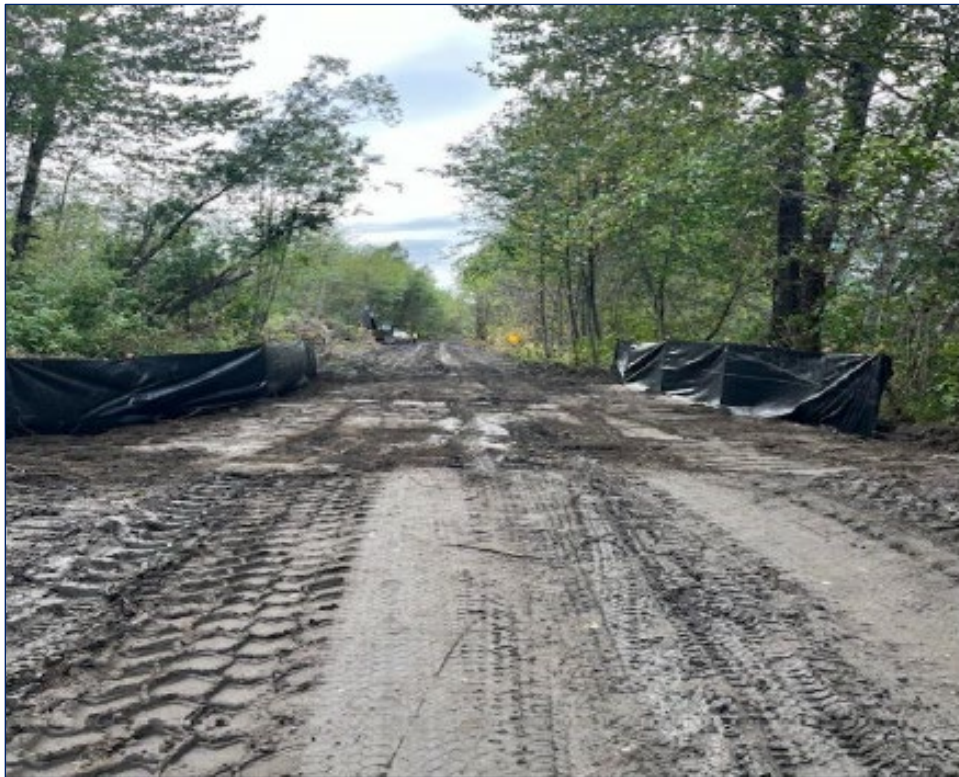
FIGURE 4-7: INSTALLING ESC MEASURES ALONG ACCESS ROAD, AUGUST 2024
