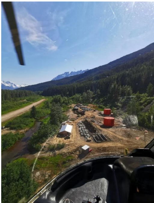
Figure 2. Aerial view of structures at the proposed site by Whitewater Creek and the temporary air strip (left)
