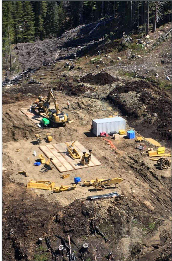
PHOTO 2-21: EQUIPMENT ASSEMBLY AT CAMP 9
