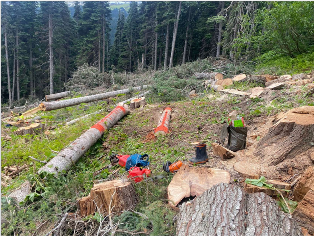
PHOTO 2-29: GROUND LEVEL DEPICTION OF MTT LAYDOWN CLEARING ACTIVITY
