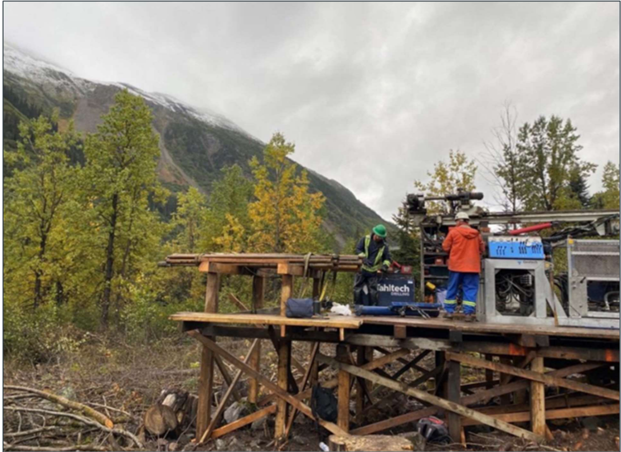
PHOTO 2-28: GEOTECHNICAL DRILL AND PAD ON THE CLEARED MTT PAD
