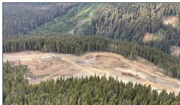
PHOTO 2-19: CAMP 9 EARTHWORKS LOOKING NORTHWEST OVER THE MITCHELL VALLEY
