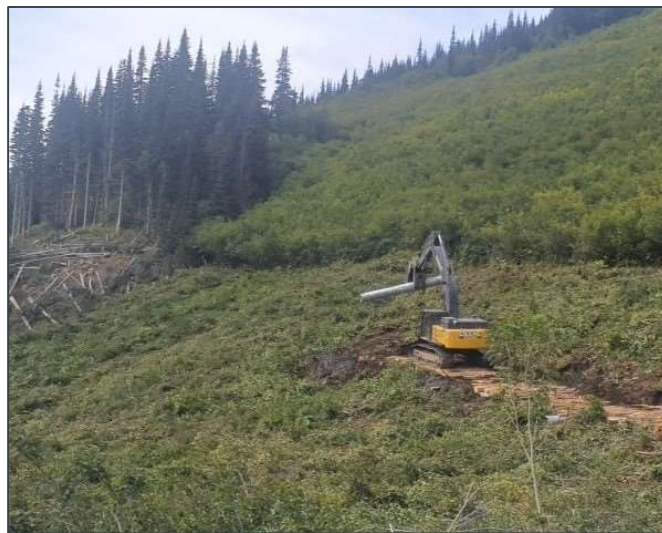
PHOTO 2-12: TREATY SADDLE ROAD CONSTRUCTION COMMENCING
