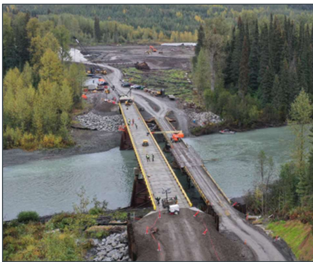
PHOTO 2-6: TEMPORARY AND PERMANENT BIRB
