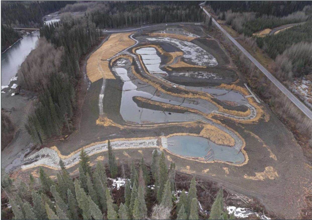
PHOTO 2-38: CONSTRUCTED GLACIER CREEK FHOP LOOKING NORTHWEST ALONG HIGHWAY 37
