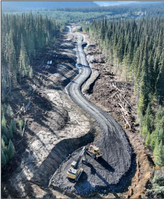
PHOTO 2-36: REPRESENTATIVE TOWER PAD CONSTRUCTION
