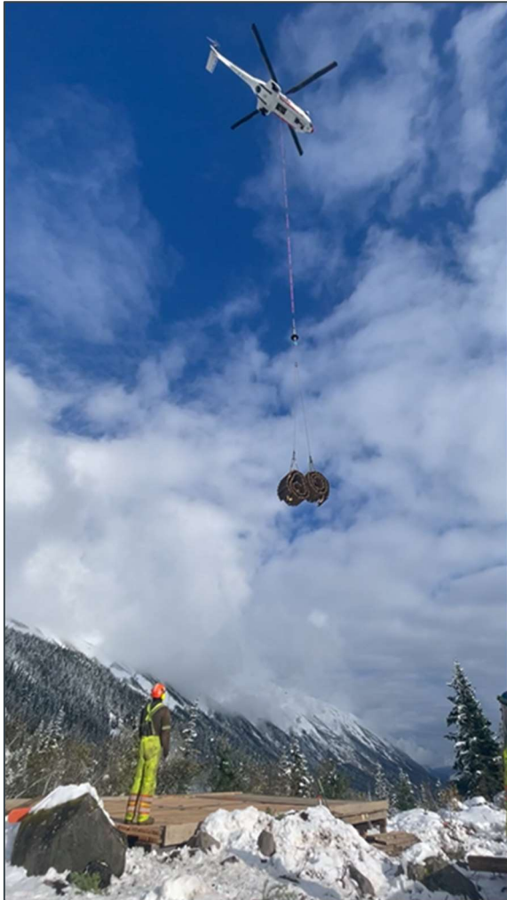
PHOTO 2-20: HEAVY LIFT OF EQUIPMENT TRACKS.
