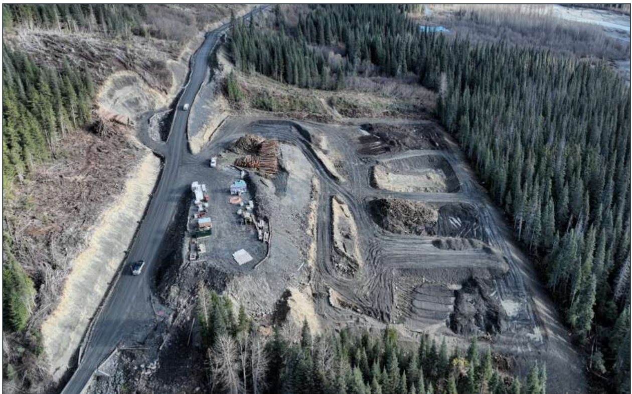
PHOTO 2-2: SOIL SPOIL PILE AREA AT KM 14 OF THE TCAR
