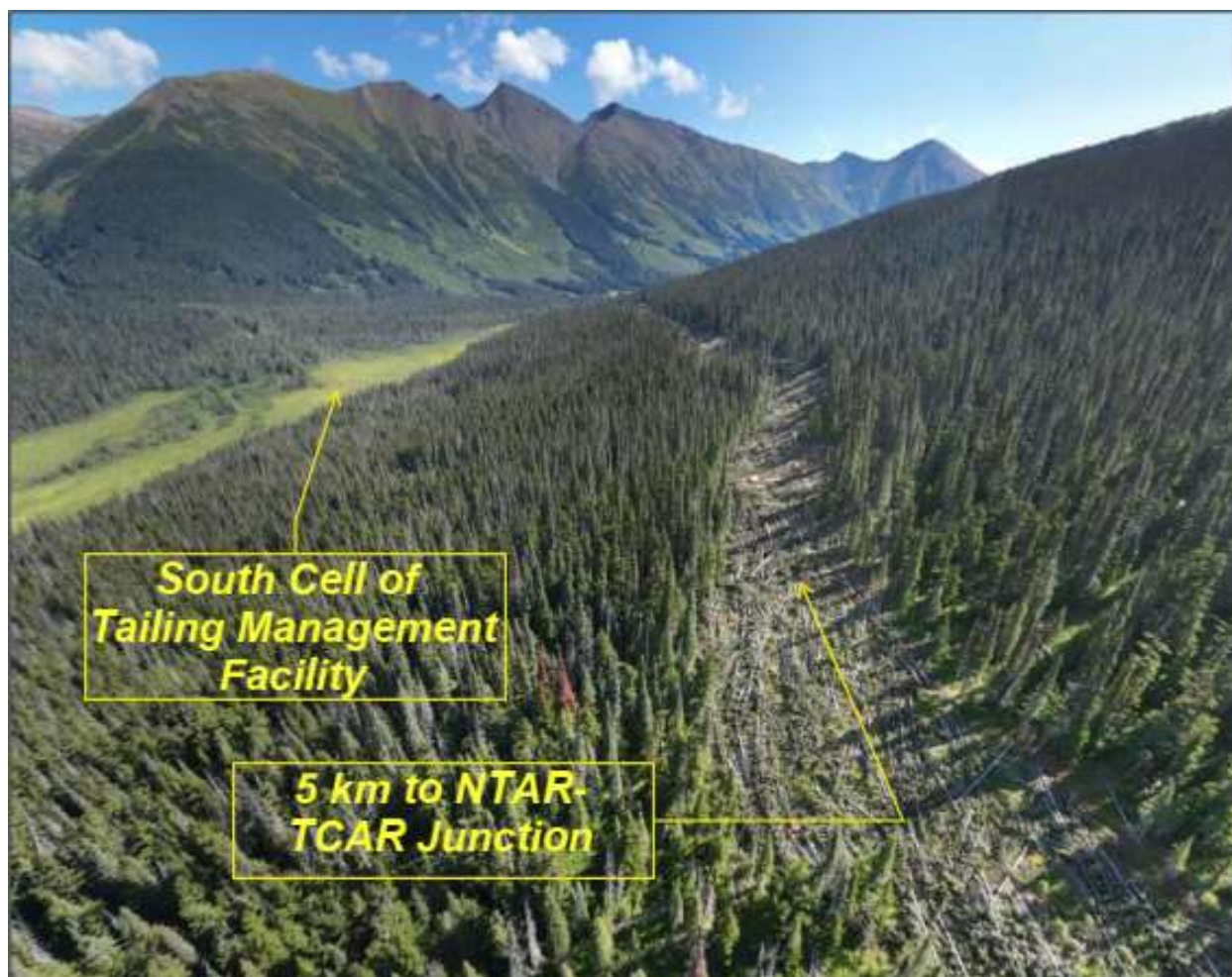
PHOTO 2-11: NTAR (~5KM FROM JUNCTION WITH TCAR) LOOKING SOUTHEAST OVER SOUTH CELL OF TAILING MANAGEMENT FACILITY.
