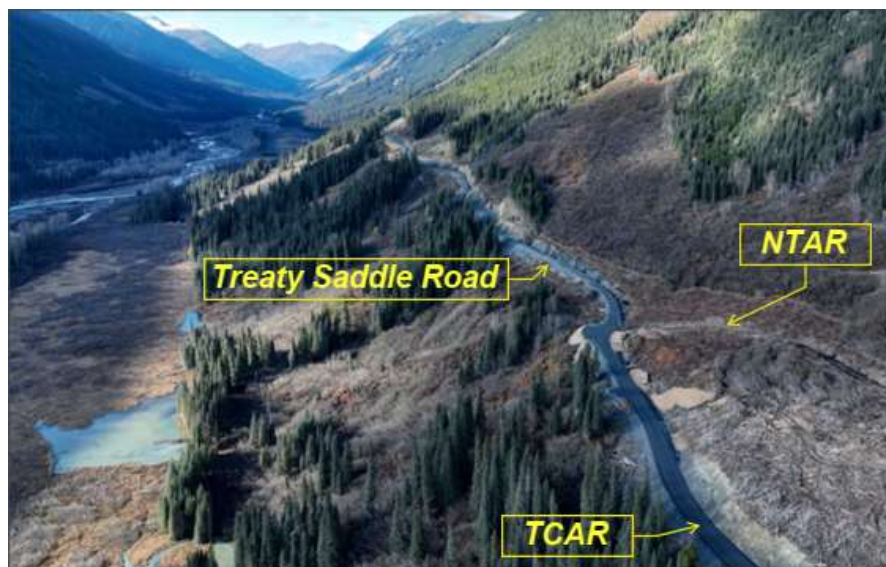
PHOTO 2-13: TREATY SADDLE ROAD WITH NTAR TREE CLEARING ON RIGHT
