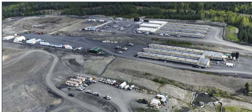
PHOTO 2-16: CAMP 11 ACCOMMODATIONS FROM SOUTHWEST CORNER OF PAD LOOKING EAST
