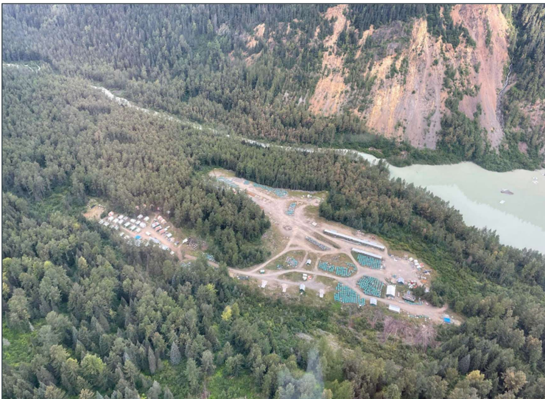
PHOTO 2-25: SULPHURETS (KSM) CAMP WITH ACCOMMODATIONS ON THE LEFT AND LAYDOWN AREAS ON THE TOP AND RIGHT
