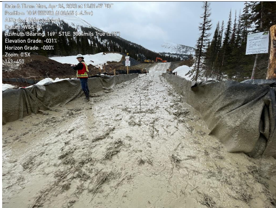
Photo 1. S2 watercourse crossing at KP 143+450. Pooling water on bridge deck.
