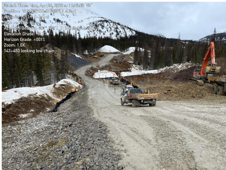
Photo 2. High chain approach to the bridge crossing at KP 143+450. Material from the travel lane flowing towards and onto the bridge deck.
