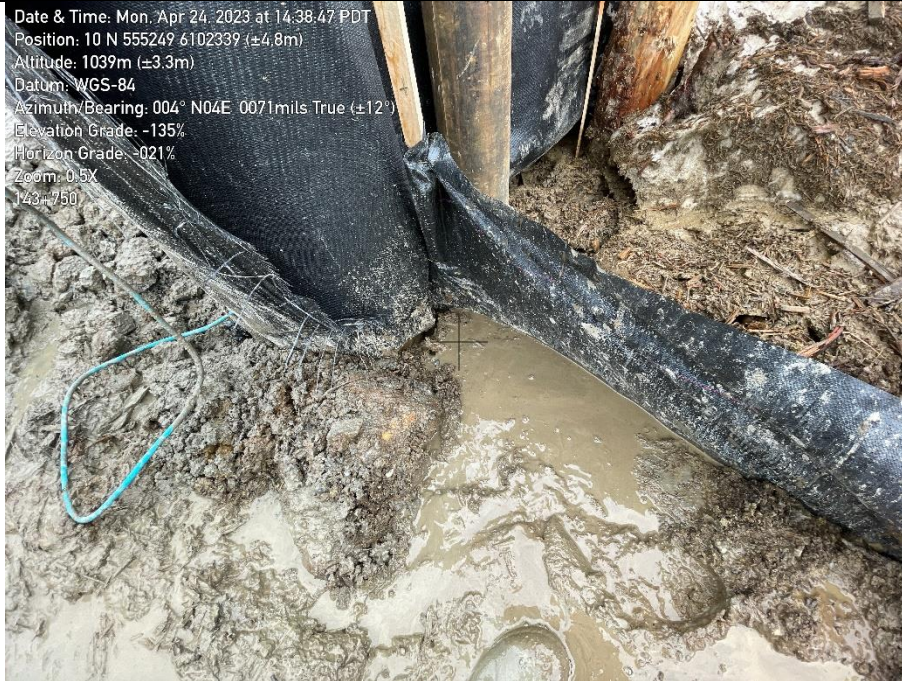
Photo 5. Sediment laden flow through measures and into watercourse at KP143+750.
