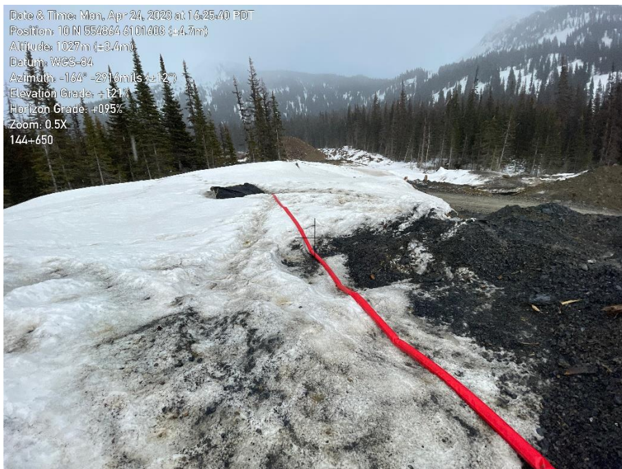
Photo 10. Second filter bag with hose primed for use.
