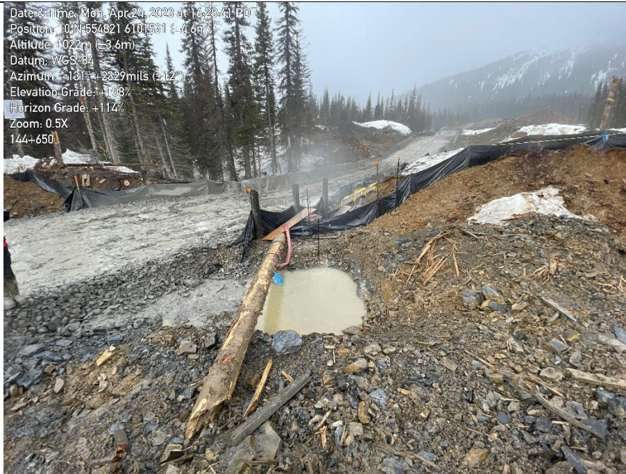
Photo 11. Sump where water is pumped into the second filter bag.
