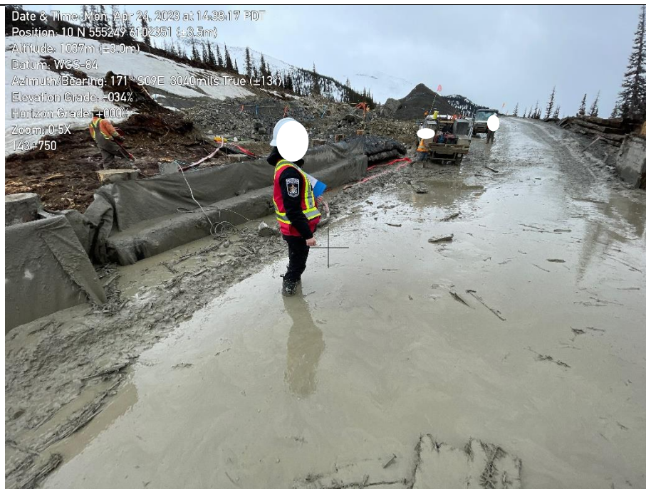
Photo 3. S4 watercourse crossing at KP 143+750. Pooling water on bridge deck.
