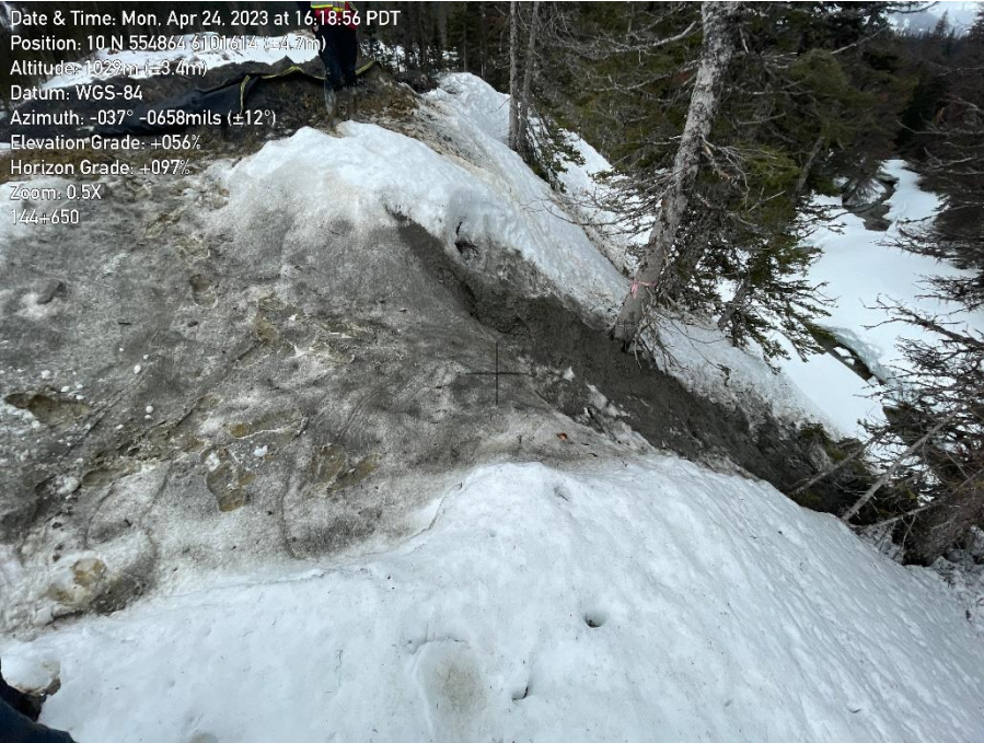
Photo 8. Deposited material from filter bag discharge at approximately KP 144+650.
