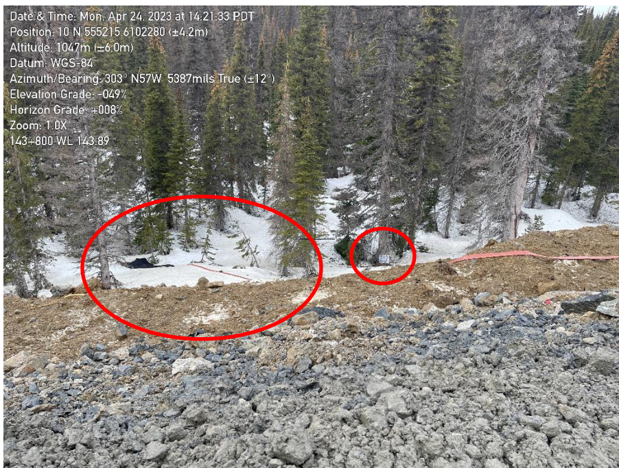
Photo 12. Filter bag set up within wetland WL-143.89. Red arrows indicate wetland identification sign and filter bag.
