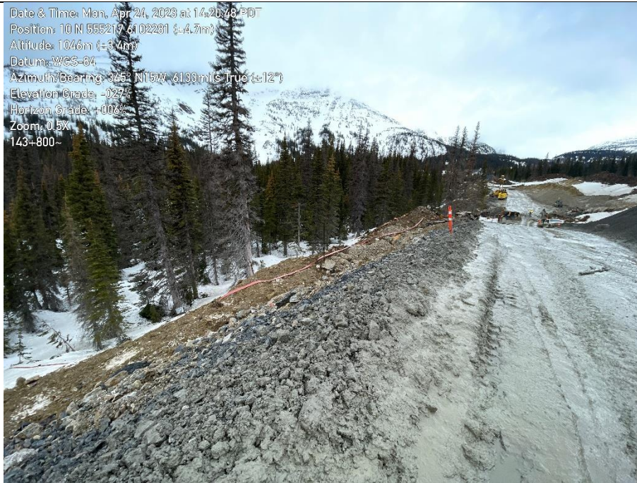
Photo 13. Discharge hose from pumping location connected to filter bag within wetland WL-143.89.
