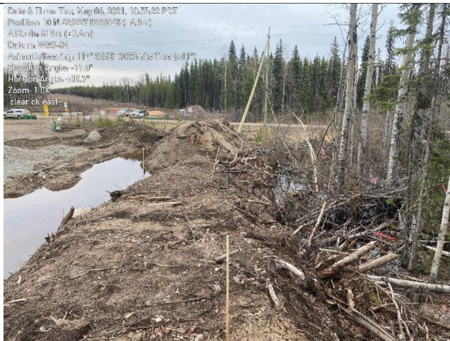
Photo 18. KP 392+282. Stockpiles on right of way within channel.
