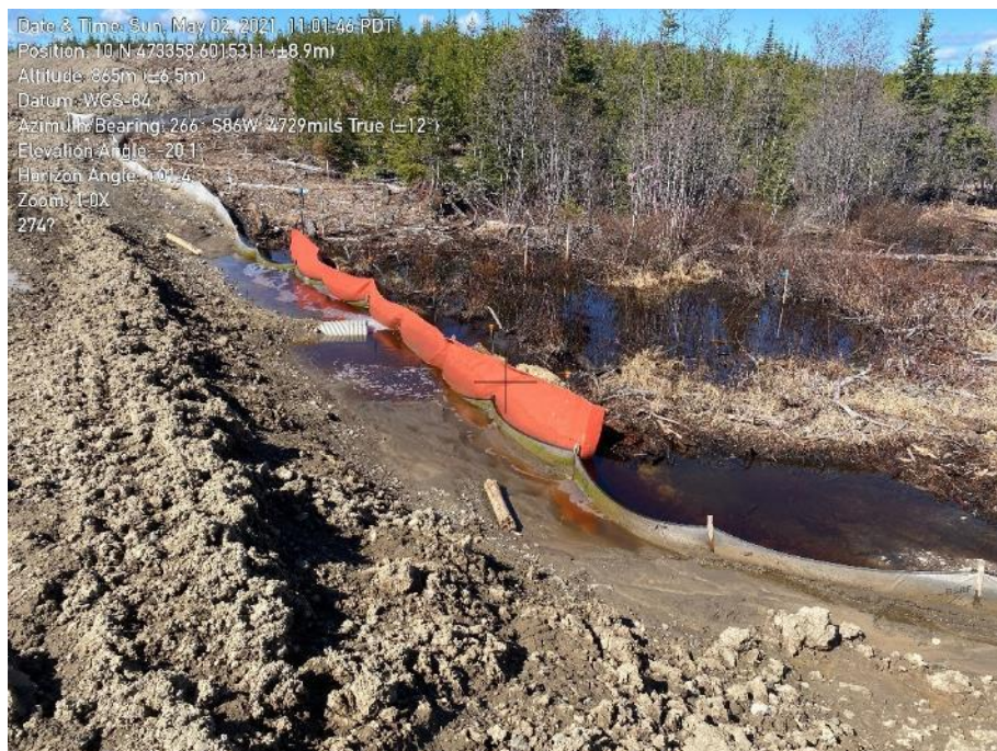
Photo 41. Non maintained ESC measure near KP 274+300.
