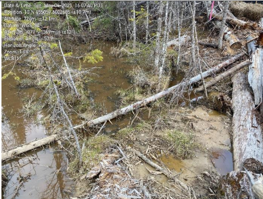
Photo 36.WL8113 at approximately KP 298+861. Sediment depositing into wetland feature.
