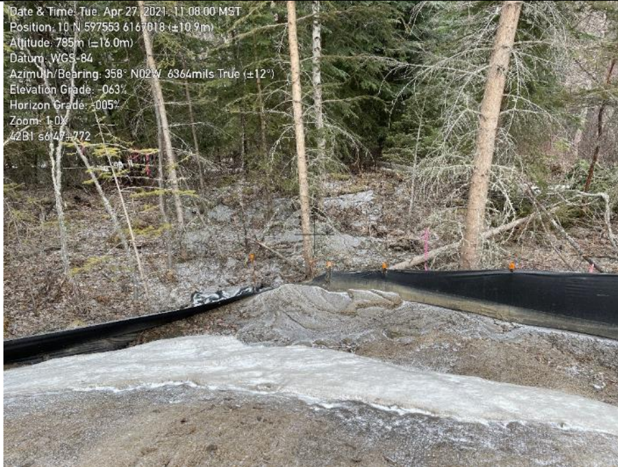
Photo 2. Section 1, watercourse 42B1, S6. Overwhelmed ESC measures with sediment leaving RoW and observed in channel downstream.
