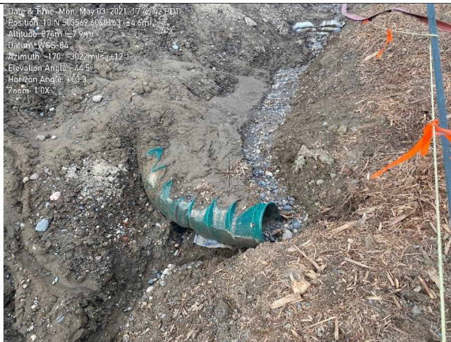
Photo 38. Example of non maintained ESC measure seen near KP 227+800.
