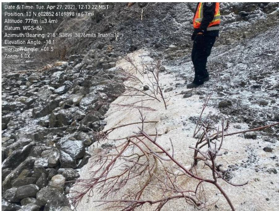
Photo 82. KP 41. Overview of planting at site. Willows not planted to depth, do not reach diameter requirement, not spaced to specification and are less than 2 – 3 m long.
