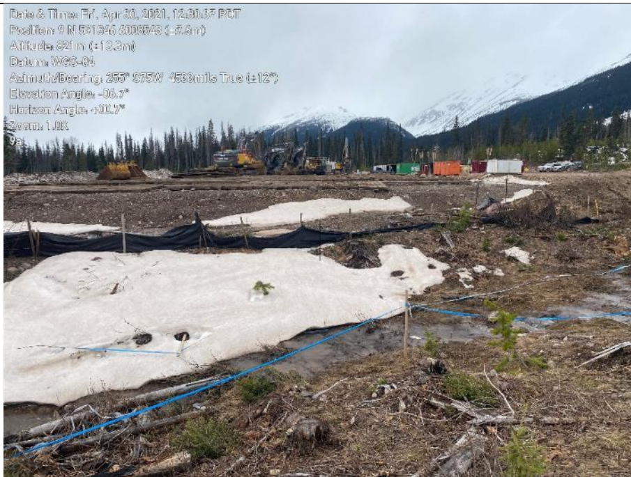
Photo 48. Failing sediment fence at Camp 9A.
