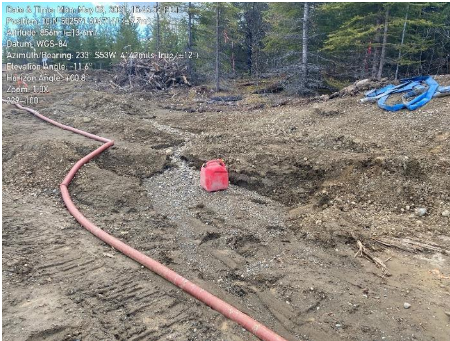
Photo 88. Approximately KP 229+100. Canister of gasoline left unattended on the right of way. Note eroded channel beneath the canister indicating flowing water recently occurred at this location.
