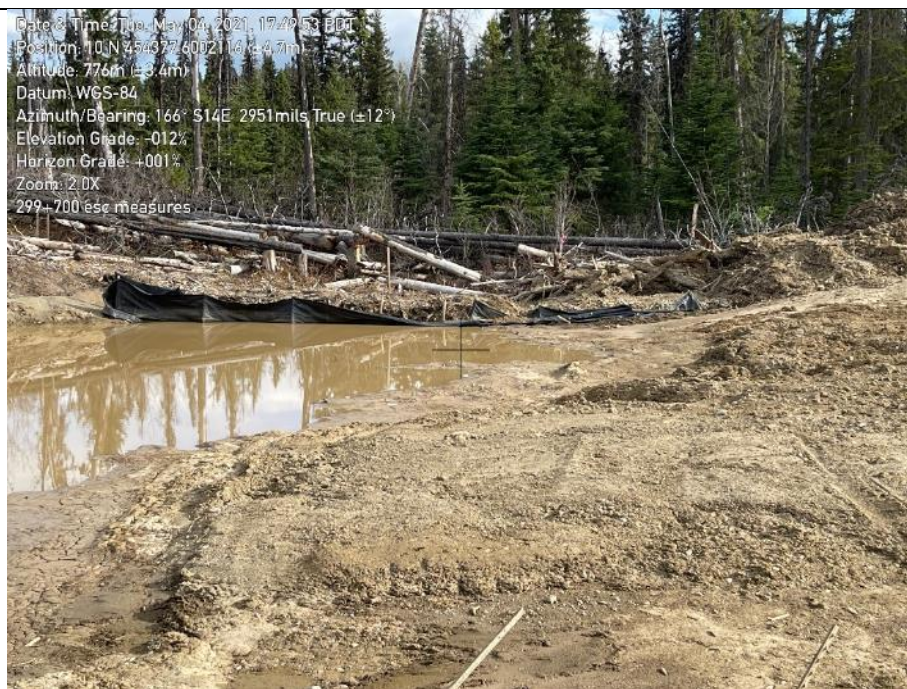
Photo 46. Approximately KP 299+700. ESC measure collapsed.
