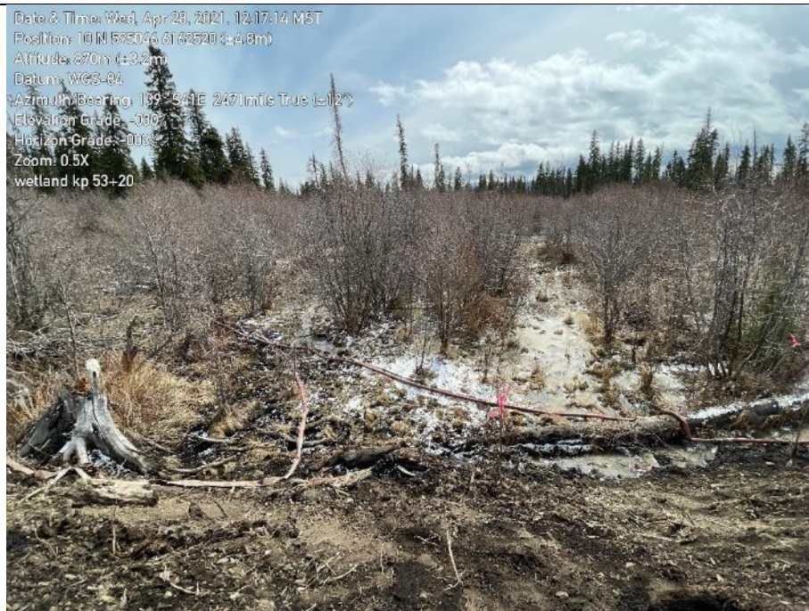
Photo 28. WL0723. Sediment laden water from filter bag draining back into wetland outside of RoW.
