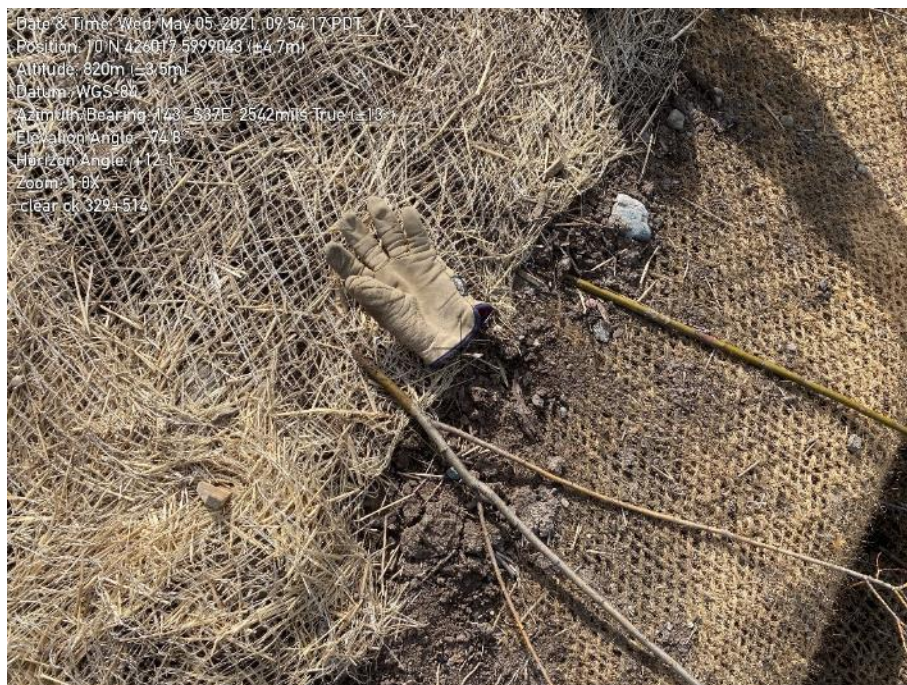
Photo 86. KP 329+300, Clear Creek. Example of depth willow stakes are planted (more than 25 cm exposed). Diameter less than 1.5 – 2.5 cm.
