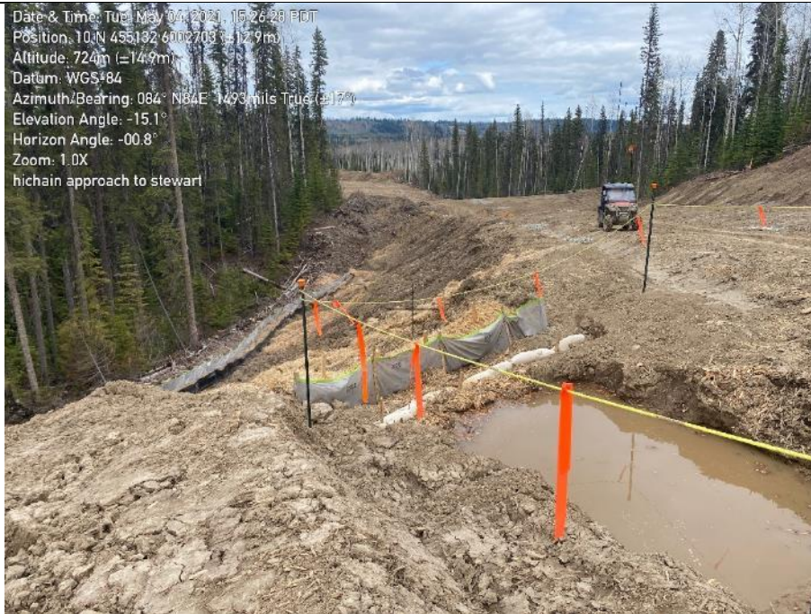
Photo 32. Wetland with no signage at roughly KP 298+700. Sediment laden water from this location left RoW and reached wetland below (WL0552).
