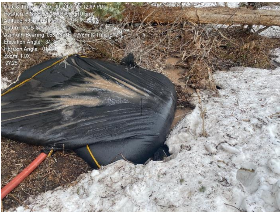
Photo 25. KP 586+800, sediment bag placed within 2 m of channel. Discharge into feature.
