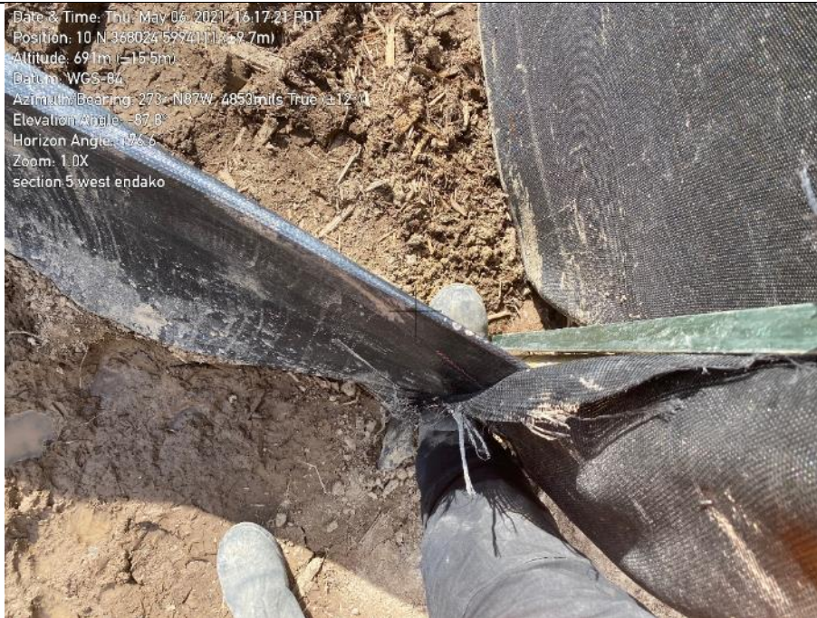
Photo 50. Approximately KP 392+400. Gap beneath sediment fence where two sections meet. Adjacent to stream crossing.
