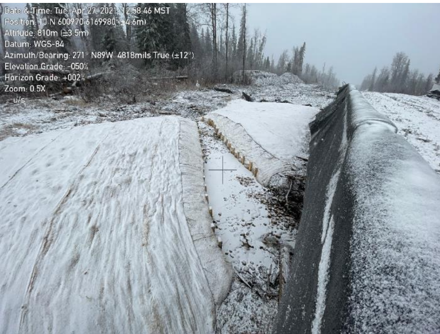
Photo 74. Watercourse UN41-30, S4. Lack of channel profile through crossing. Potential barrier to fish passage.
