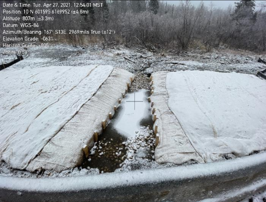
Photo 73. Watercourse UN41-34, S4. Lack of channel profile through crossing. Potential barrier to fish passage.
