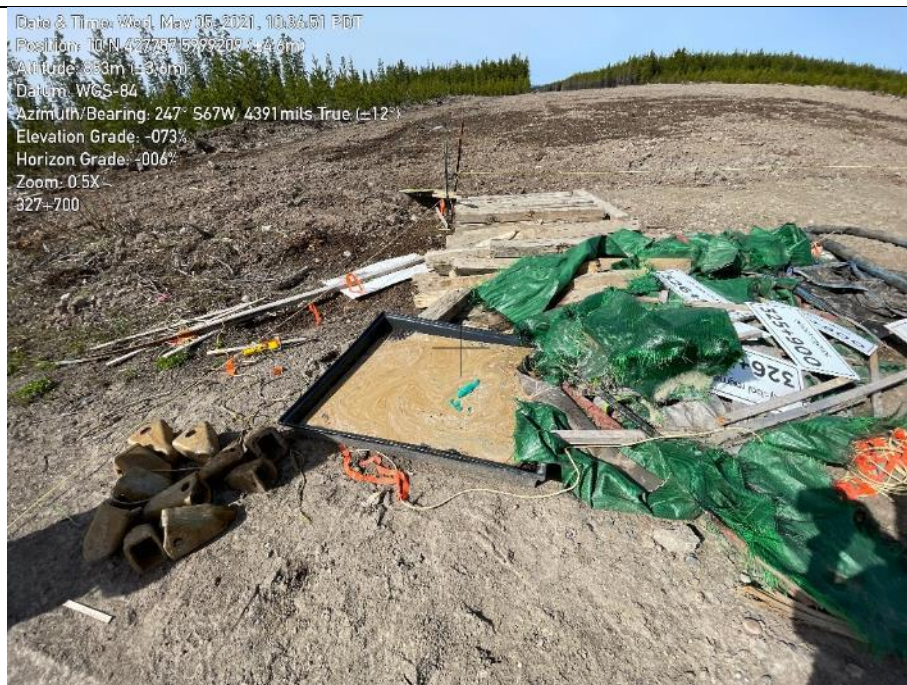
Photo 95. Secondary containment near capacity with oily sheen observed at KP327+700.
