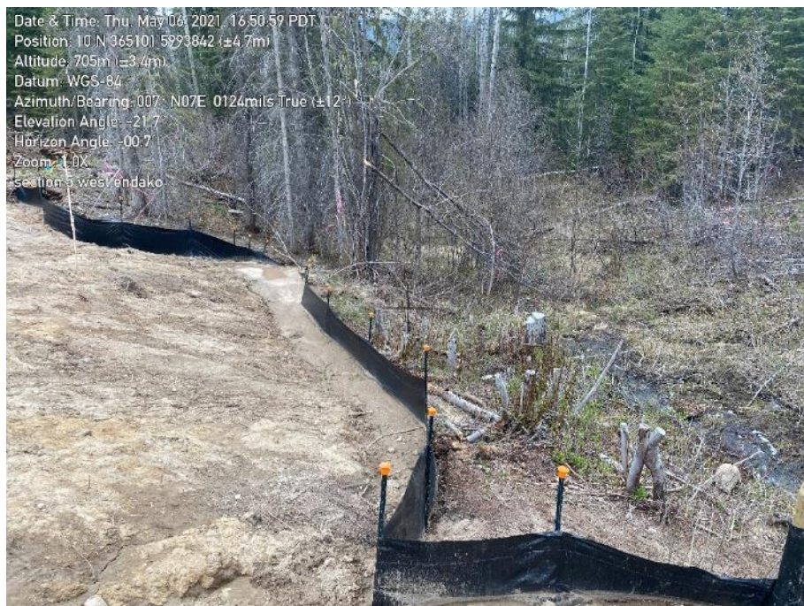
Photo 21. KP 395+542 (S6). Overwhelmed / not maintained ESC measures.
