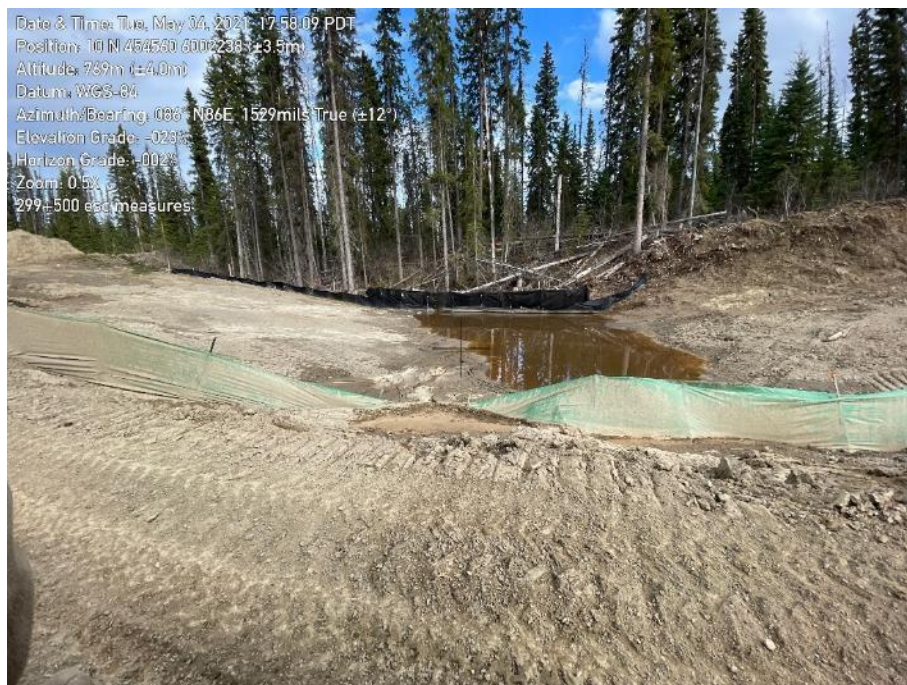
Photo 47. Approximately KP 299+500. ESC measure overwhelmed and collapsed.
