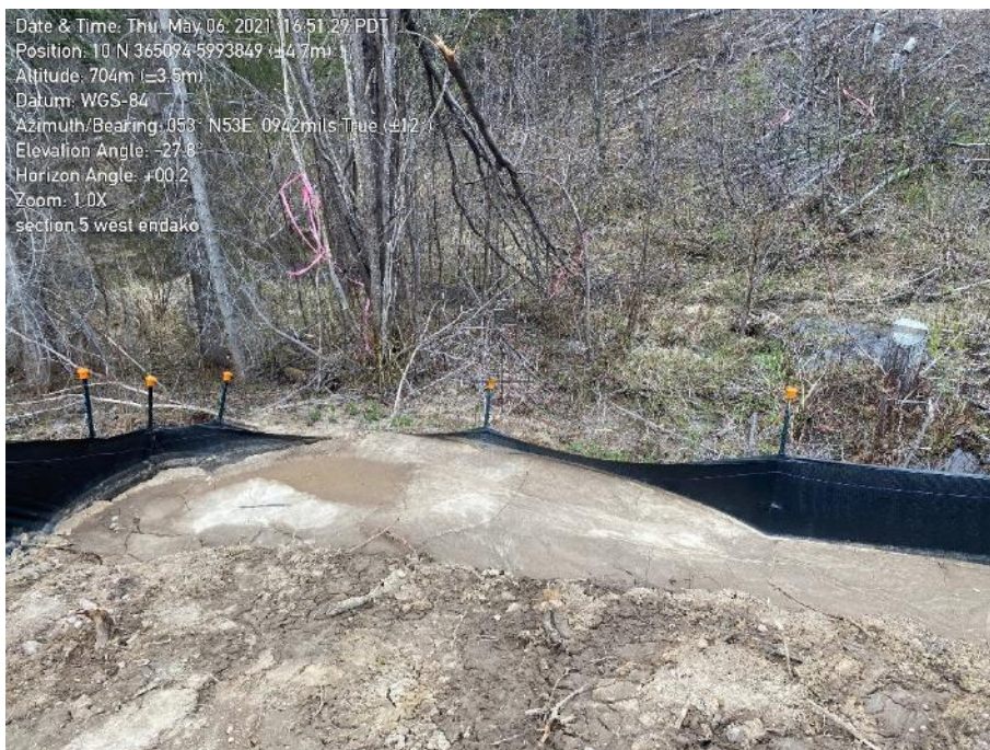
Photo 49. Failing ESC measure at approximately KP 395+550. Lead to sediment discharging into stream feature.
