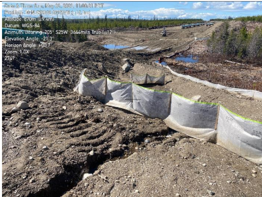
Photo 40. Non maintained ESC measure near KP 274+300. Erosion taking place beneath the measure.
