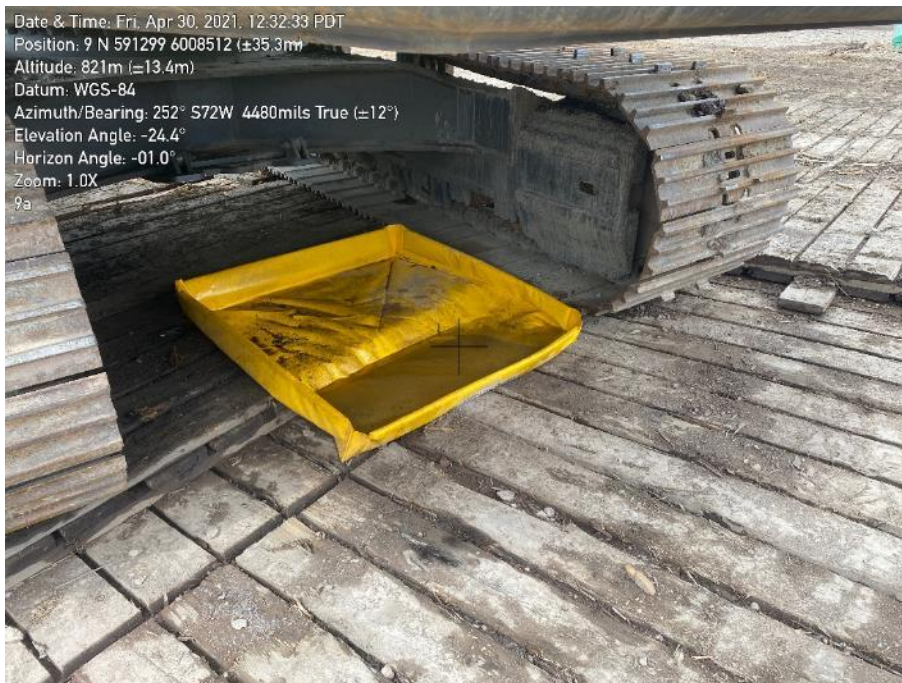
Photo 94. Secondary containment on angle and water at risk of leaving containment - Camp 9A.
