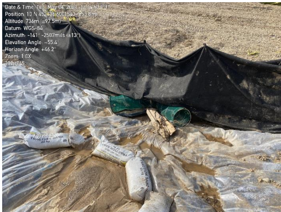
Photo 45. KP 302+045. ESC measures installed in front of culvert inlet. Measures observed to require maintenance.
