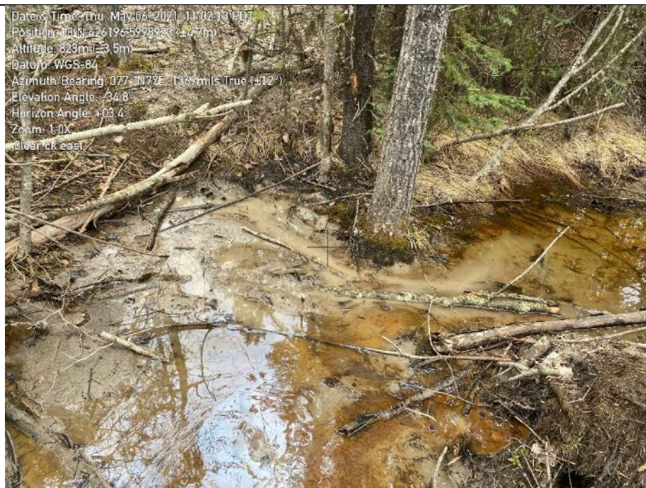
Photo 20. KP 392+282. Sediment from filter bag entering water feature.
