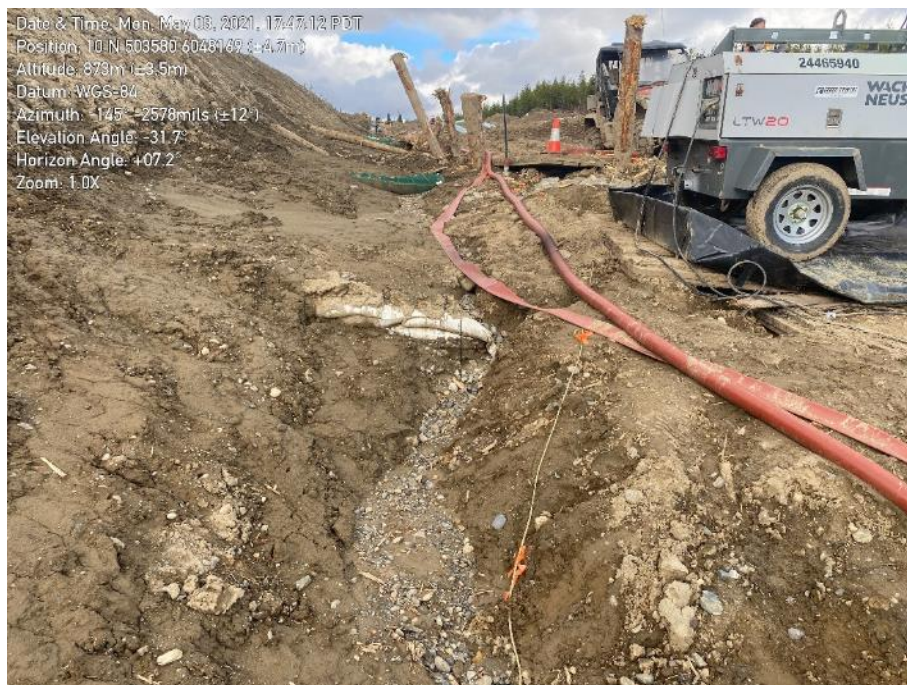
Photo 39. Example of non maintained ESC measure seen near KP 227+800.
