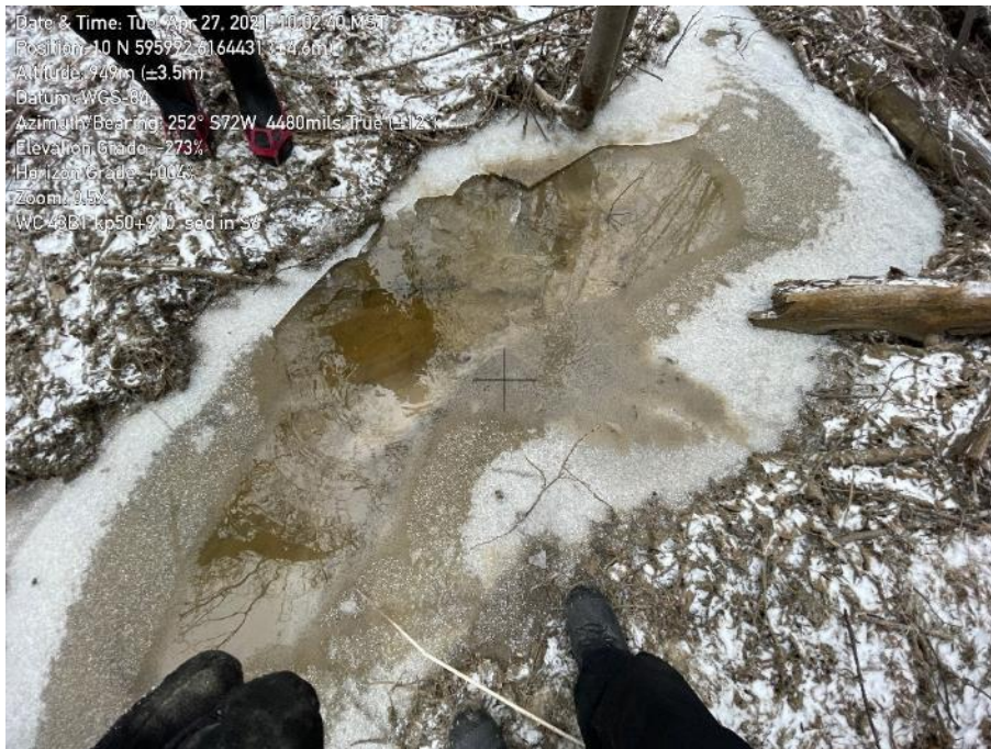
Photo 1. Section 1, watercourse 43B1, S6. Sediment laden water overtopped sediment fence and observed in channel downstream of crossing.
