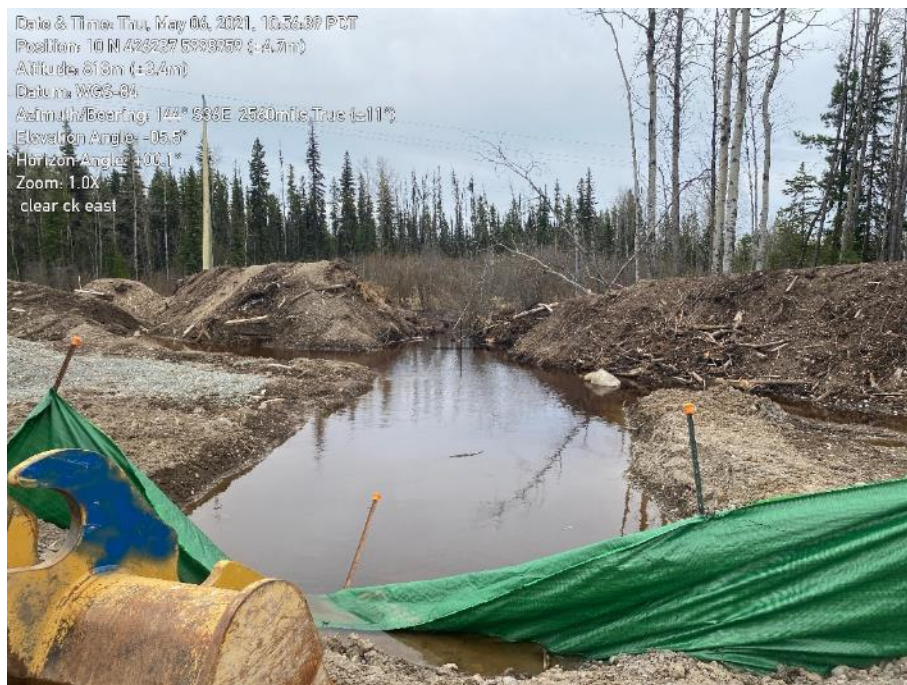
Photo 17. KP 329+282. Looking downstream from culvert outlet on right of way. Stockpiles on right of way with no mitigation measures.
