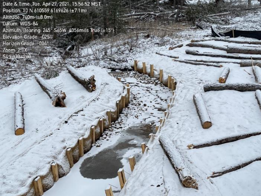
Photo 78. KP33+260, unknown watercourse number. Lack of channel profile through crossing. Potential barrier to fish passage.
