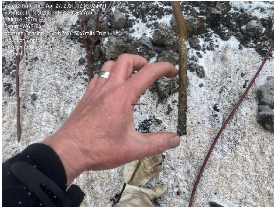
Photo 81. KP 41. Example of the observed planted depth of willow stakes. More than 25 cm left exposed after planting.
