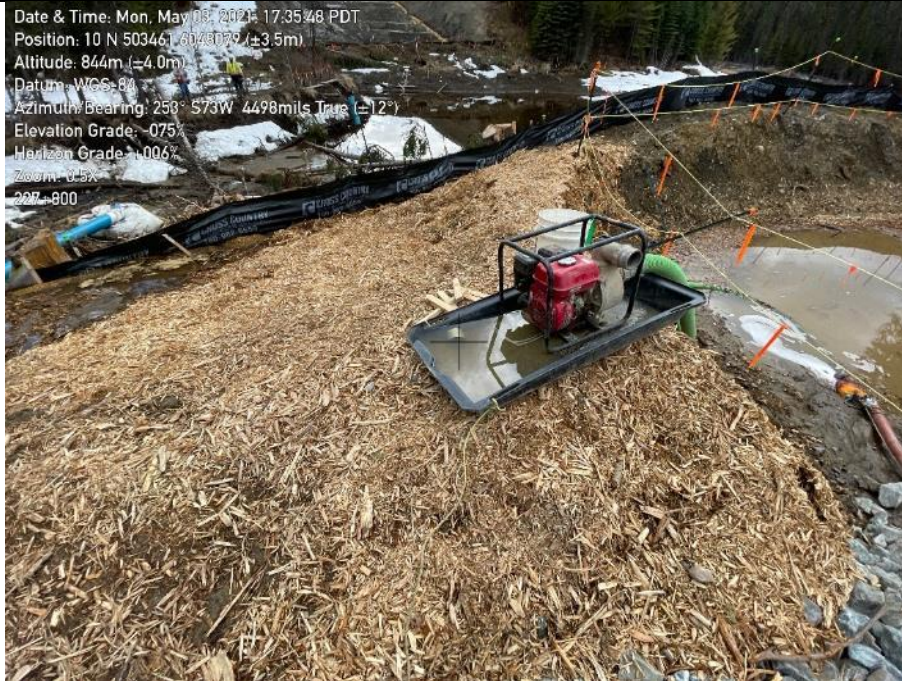
Photo 89. At capacity secondary containment within 100 m of watercourse at approximately KP 227+746. Water leaving containment structure.
