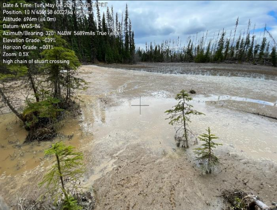
Photo 34. Wetland with no signage at roughly KP 298+700. Sediment laden water and sediment deposited in wetland (WL0552).
