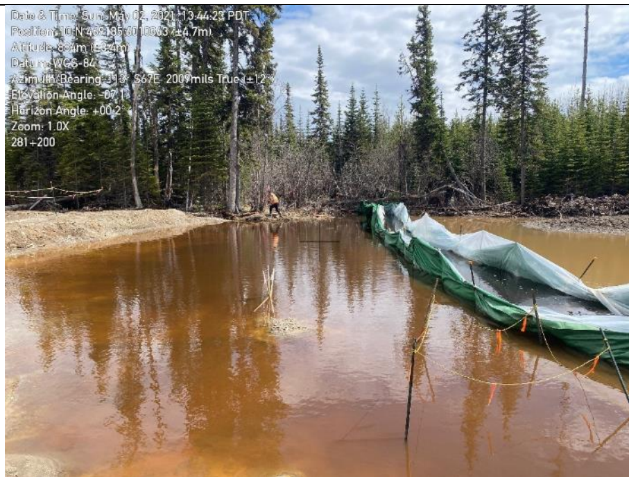
Photo 14. KP281+200. Water from RoW flowing into feature around the flume both upstream and downstream of the measure.
