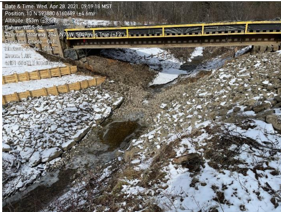
Photo 71: Watercourse 47B1, S3. Shallow flow through reconstructed channel. Potential barrier to fish passage.
