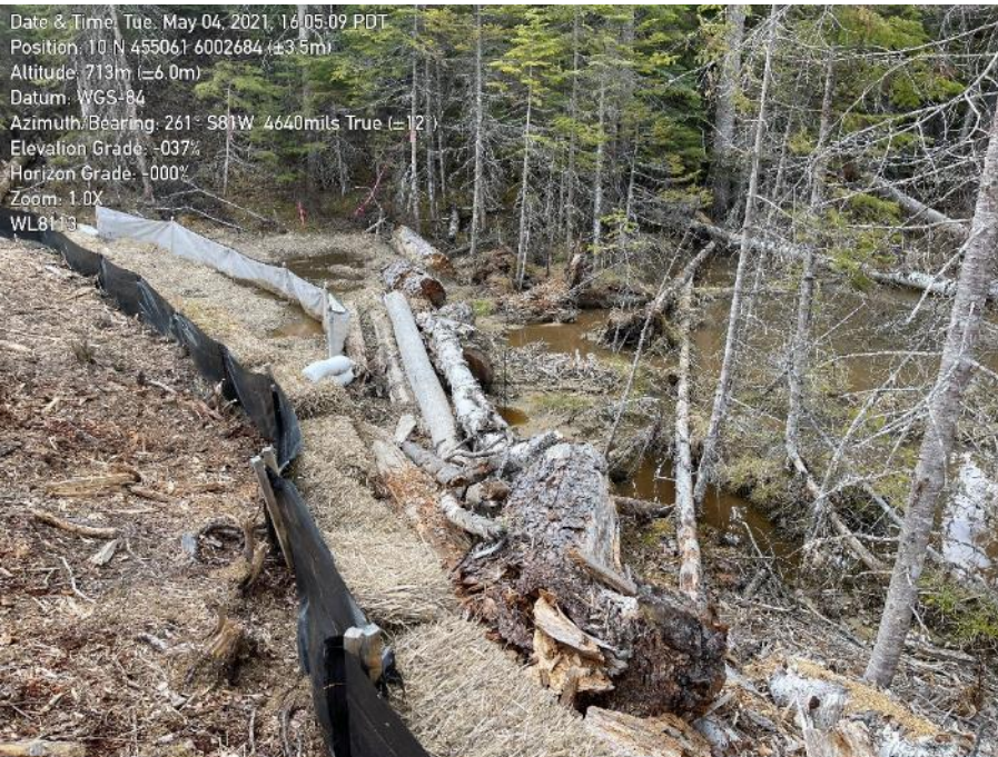
Photo 35. WL8113 at approximately KP 298+861. Sediment laden water passing ESC measures and entering wetland.
