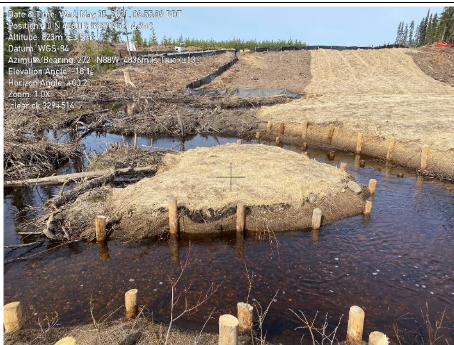
Photo 87. KP 329+300, Clear Creek. Willows not planted at one stem per 15 cm.
