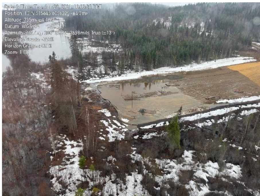
Photo 5: Section 3, Crooked River. High chain approach slopes towards Crooked River. Stripping into naturally occurring flood plain within the Crooked River. Project related exposed surfaces and sediment laden water mixing with Crooked River flows.
