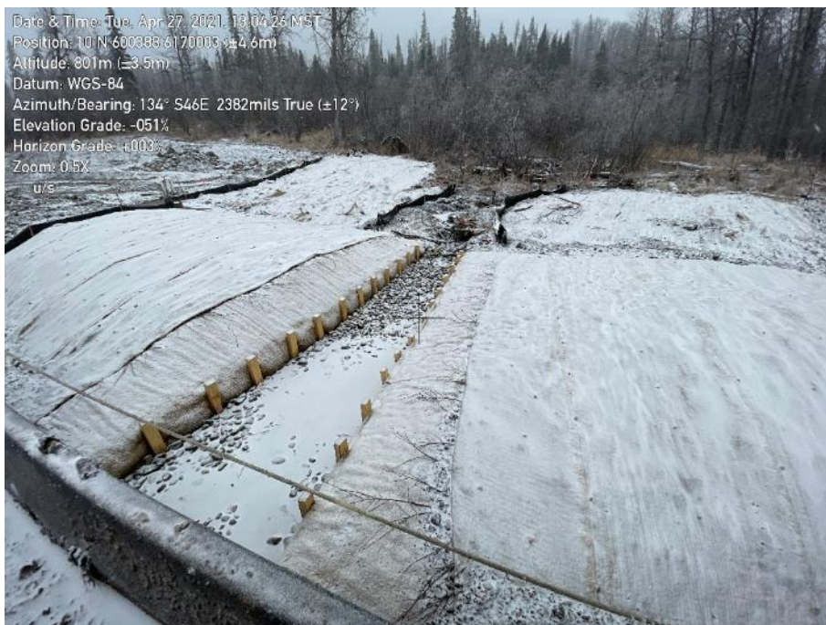
Photo 76. Watercourse UN41-28, S4. Lack of channel profile through crossing. Potential barrier to fish passage.
