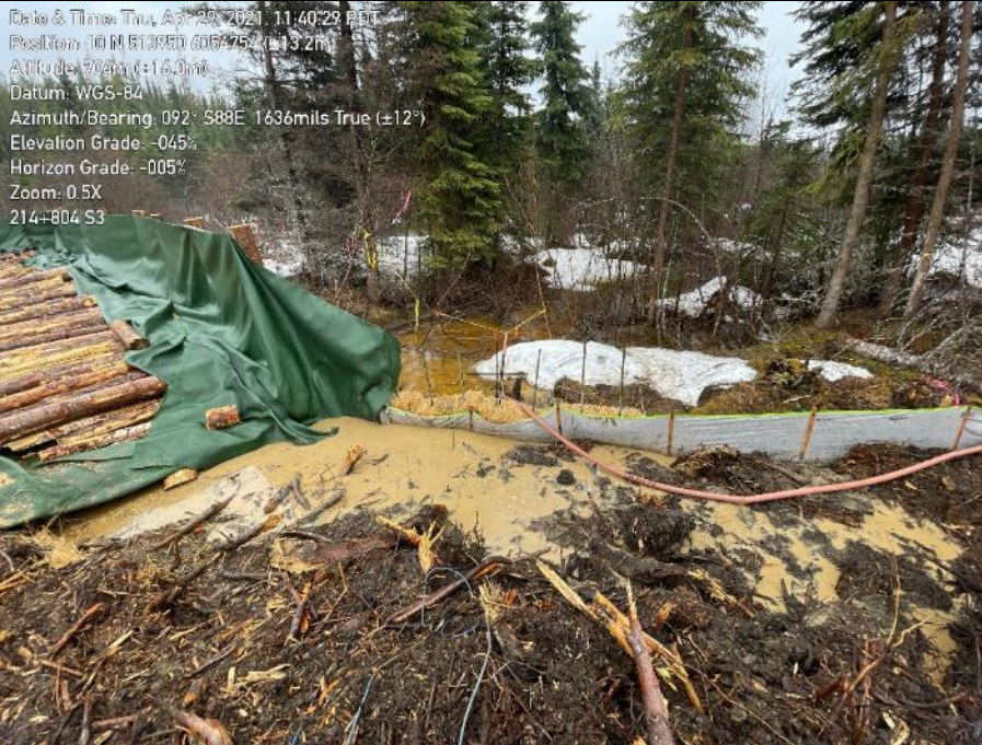
Photo 6. Section 3, approximately KP214+804, S3. Sediment laden water leaving RoW and entering channel.
