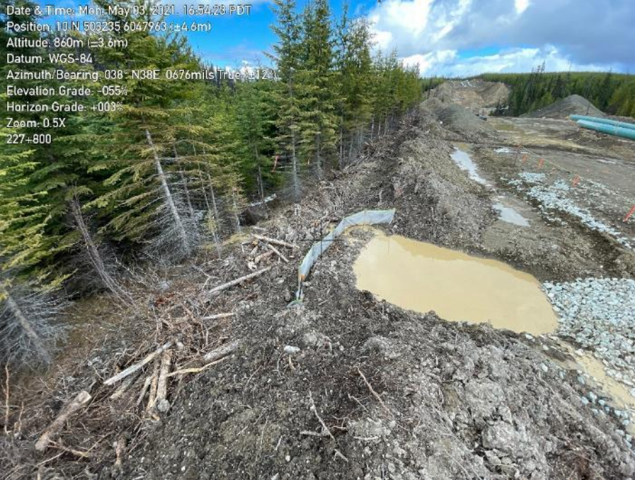
Photo 30. Sediment leaving right of way and draining towards wetland WL11553 near KP227+733.
