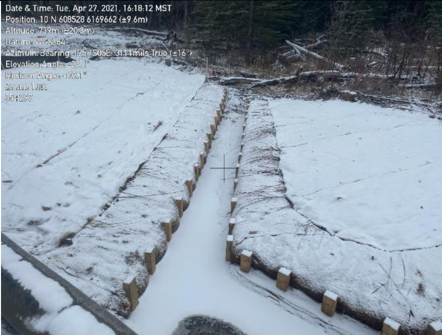
Photo 83. KP35+297. Overview of willows at site. Willows less than 2 – 3 m long, not planted to depth requirement, spacing not one stem per 15 cm.
