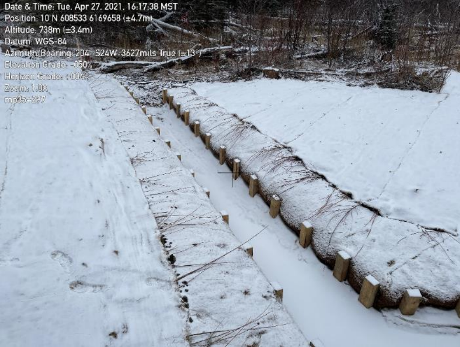
Photo 77. Watercourse UN42-22, S3. Lack of channel profile through crossing. Potential barrier to fish passage.
