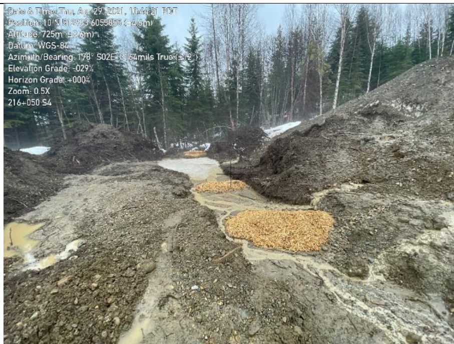
Photo 10. Water bar on high chain side of KP216+050 (S4). From RoW looking at forest.
