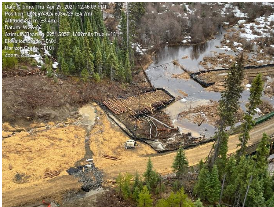
Photo 15. KP 244+510, watercourse WC272 (S3). Water from RoW overwhelming sump and flowing into stream feature.
