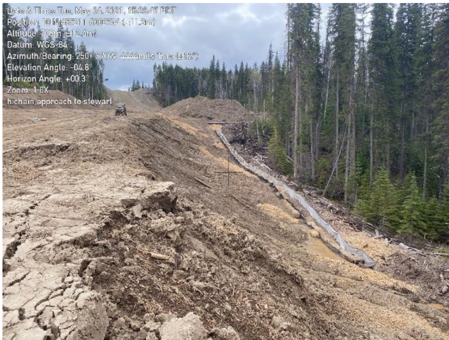
Photo 33. Wetland with no signage at roughly KP 298+700. Sediment laden water from this location left RoW and reached wetland below (WL0552).
