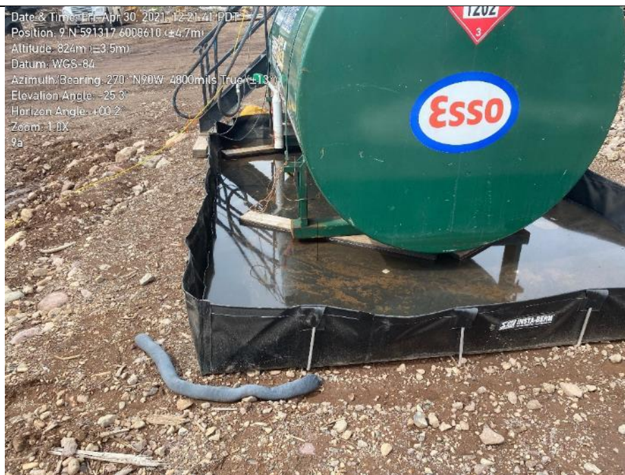
Photo 91. Above ground fuel storage with water accumulating in secondary containment - Camp 9A.
