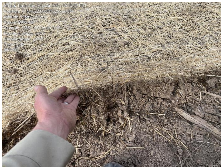
Photo 43. KP 301+900, loose erosion control blanket with limit staples/stakes.
