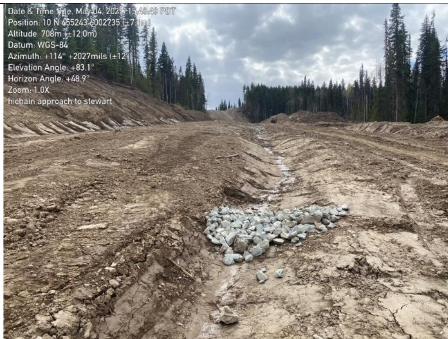
Photo 42. KP 299+100. Coarse material used for check dam construction. Flow beneath the check dam. Large spacing between check dams.
