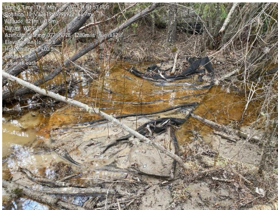
Photo 19. KP392+282. Filter bag potentially placed within WL11248 downstream of right of way. Sediment mobilized into NCD feature with direct connection to Clear Creek.
