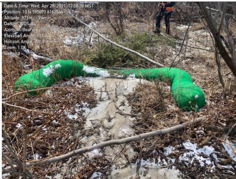
Photo 52. Erosion and flow beneath ESC measure.
