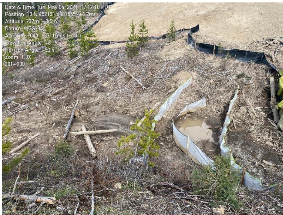
Photo 44. KP 302+045. ESC measures installed across channel. Measures full and require maintenance.
