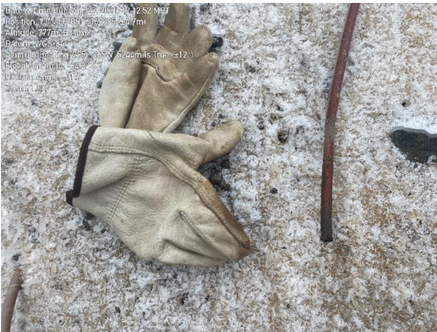
Photo 80. KP 41. Example of willow stake diameter (less than 1.5-2.5 cm diameter).
