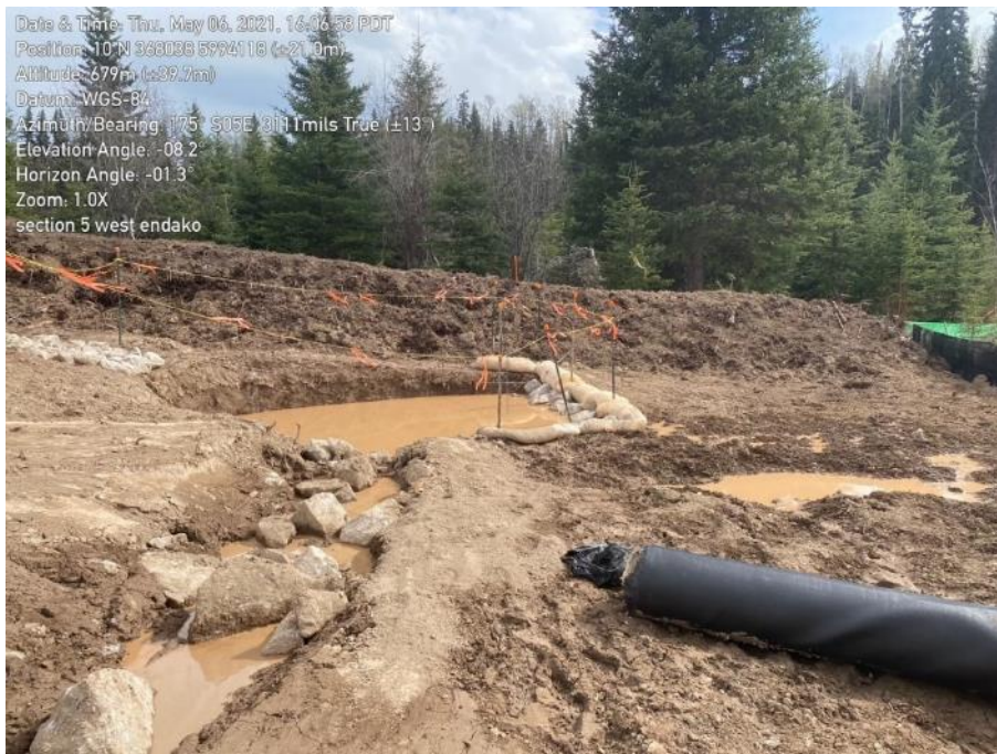
Photo 51. Example of a full sump with sediment laden water overtopping banks.
