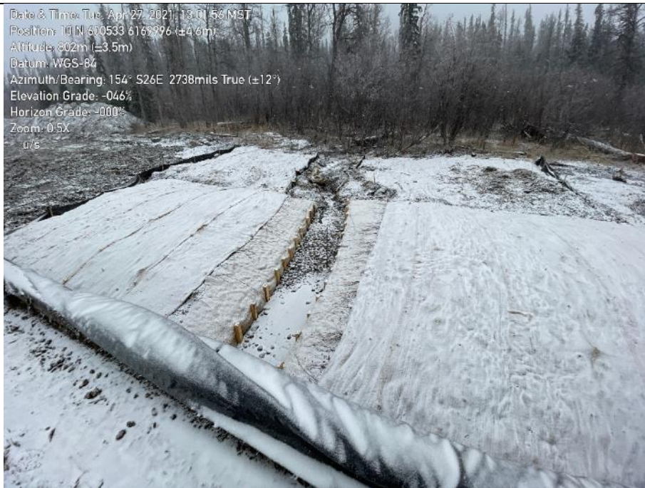
Photo 75. Watercourse UN41-29, S4. Lack of channel profile through crossing. Potential barrier to fish passage.
