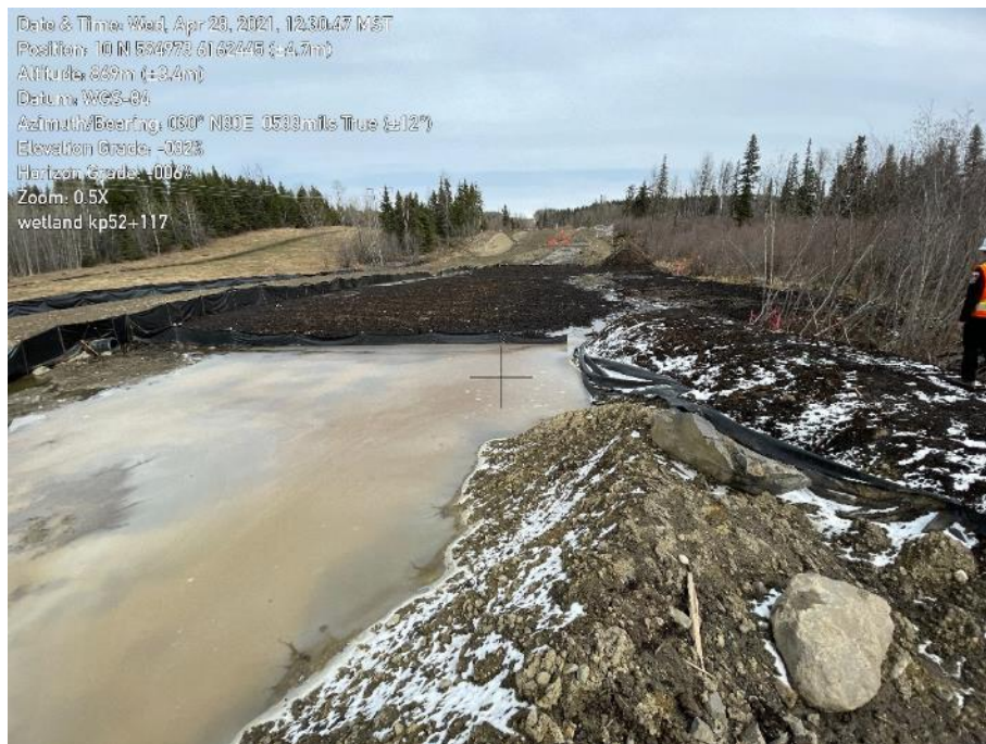
Photo 29. WL0723. Sediment laden water from RoW flowing into wetland.
