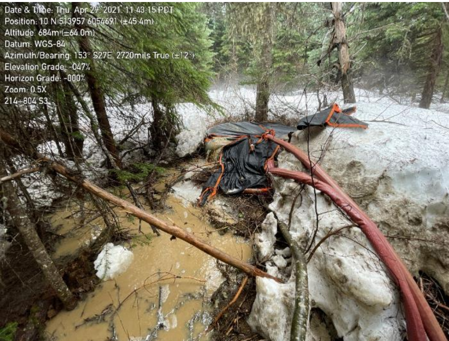
Photo 7. Section 3, approximately KP214+804, S3 High chain sump draining through filter bag. Water from bag then flows back towards and into S3 stream.
