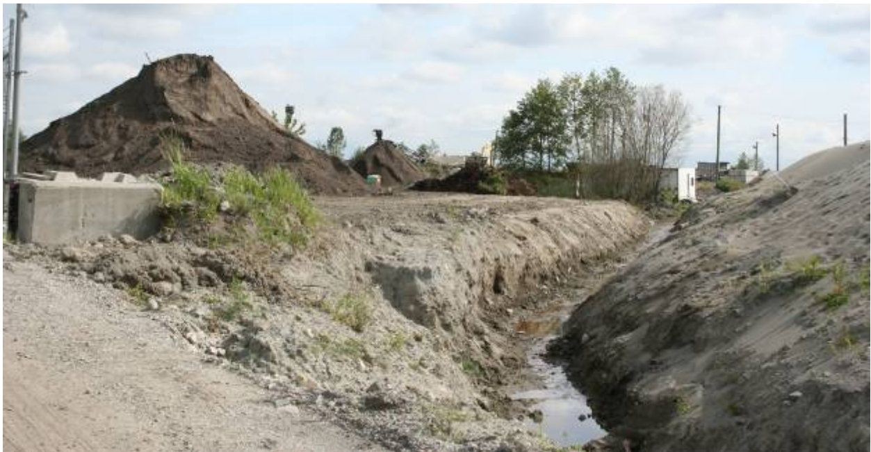
Photo 2.7.6 View east along drainage channel between north toe of pre-load and ACME Landfill & Peat Ltd. (the proposed fuel receiving facility site) (June 22, 2010)
