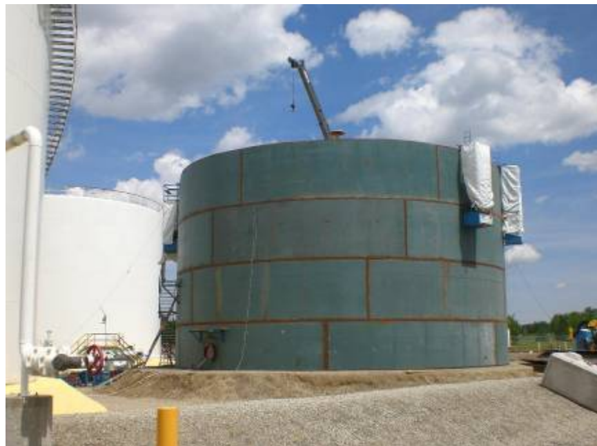
Photo 2.4.7 Typical Tank Construction (2)
