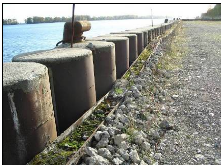
Photo 2.4.2 View Southwest (Downstream) along the Existing Bulkhead Wall
