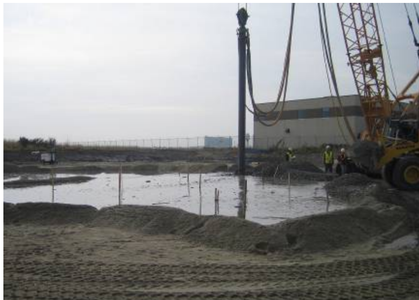
Photo 2.4.3 Typical Vibro-replacement Method of Ground Improvement
