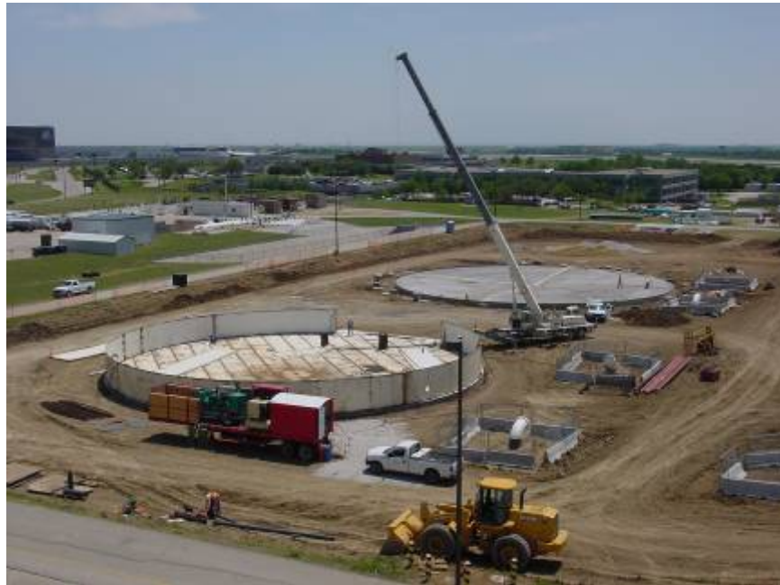
Photo 2.4.6 Typical Tank Construction
