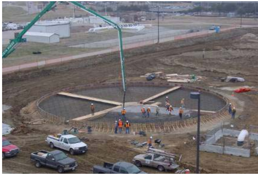
Photo 2.4.4 Typical Tank Foundation Installation
