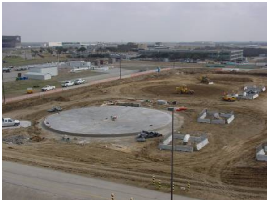
Photo 2.4.5 Typical Completed Tank Foundation
