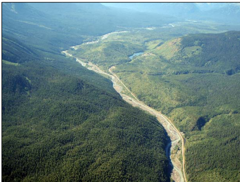
Figure 4. View downstream on Ningunsaw River from above Alger Creek showing Highway #37 and Echo Lake.
